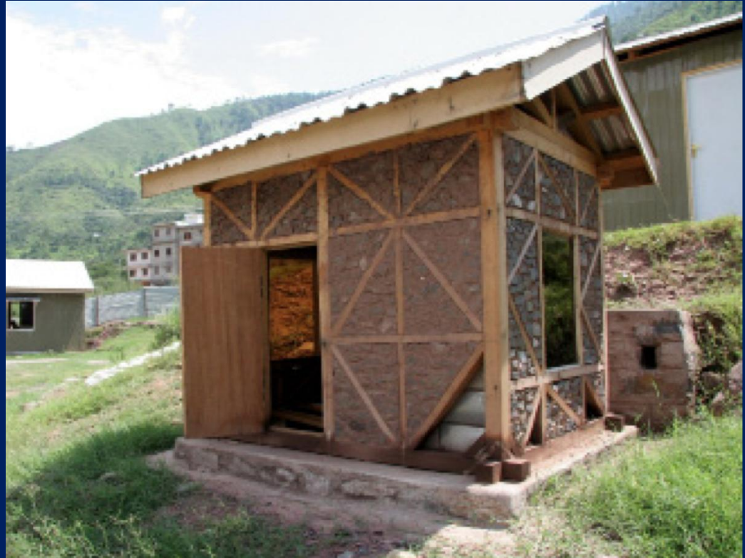
Half-timber and stone infill hut in Pakistan © UN-Habitat
