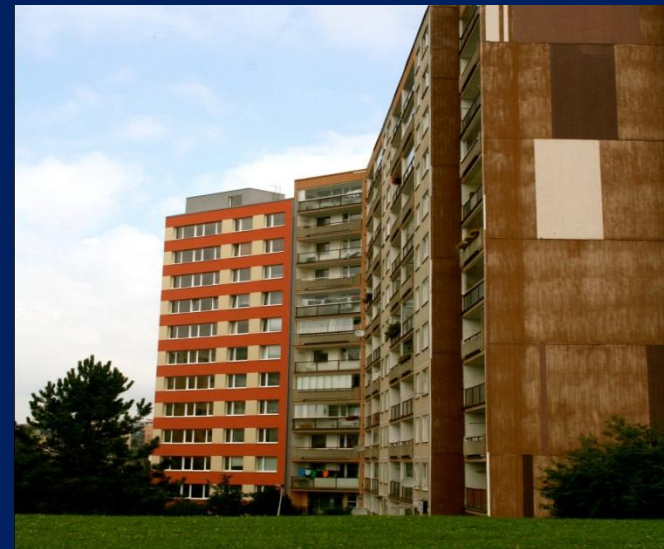
Building undergoing retrofitting in Czech Republic © UN-Habitat
