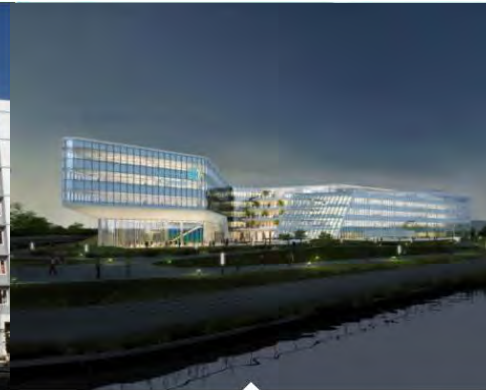
Johnson Controls HQ Asia Pacific 📍 China
