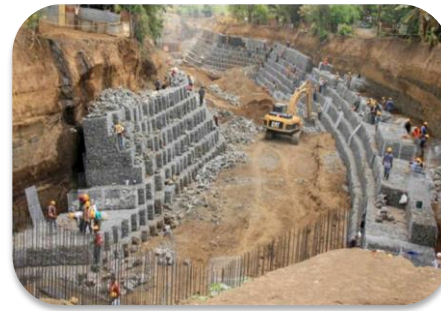
Expansion of drainage systems
