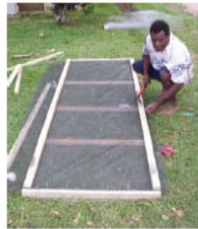
2. Stretching the chicken wire on the frame
