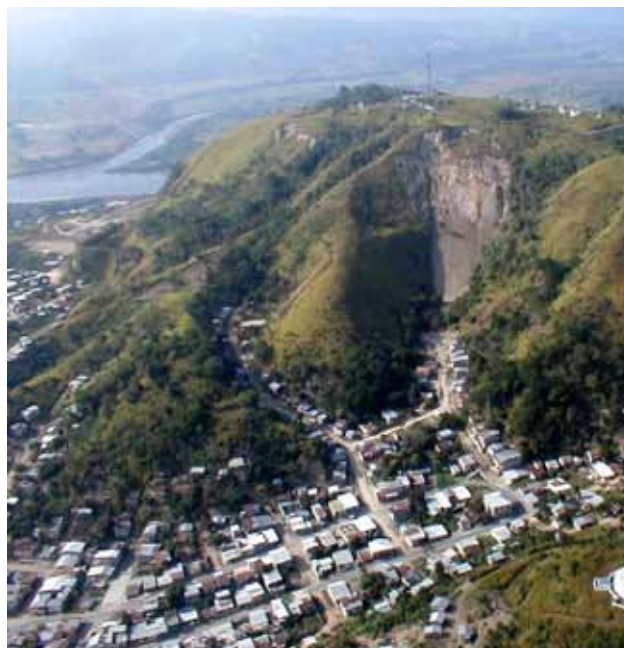
Settlements on the hills are prone to landslide. Photo © UN-HABITAT
