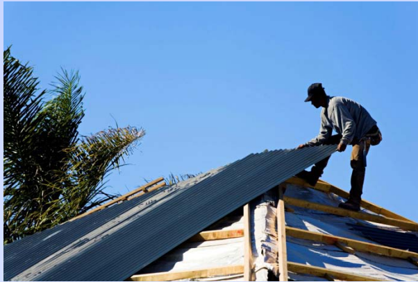
Improvements in roofing, Jamaica
