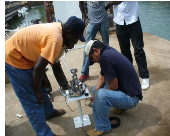
Installing Tide gauge
