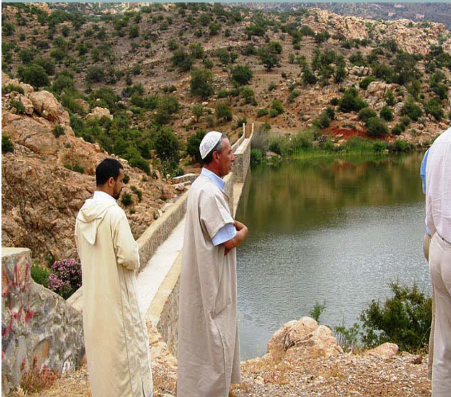
Small Dam in Souss S. Morocco
